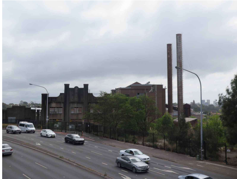
Figure 14 – View looking northeast from the Victoria Road overpass near Lilyfield Road to White Bay Power Station, a heritage item of State significance, located north of the Glebe Island Silos (Source: NBR SARCHITECTURE, October 2017)
