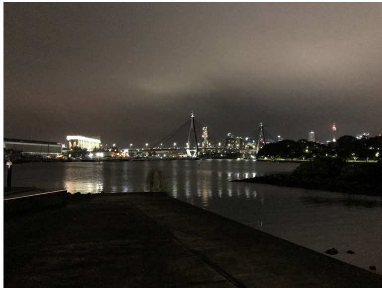
Figure 24 – Night view of the Silos from Jubilee Park alongside the other city lights. ( NBR SARCHITECTURE June 2021)
