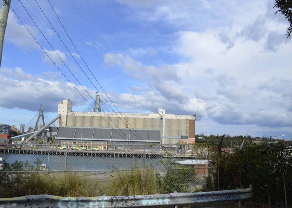
View 41: From adjacent to the public park at the corner of Mansfield St and Batty St, Rozelle. Photography by GroupGSA
