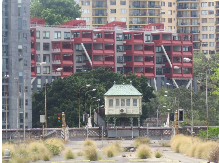
Figure 31 – View east from Somerville Road to Glebe Island Bridge, a heritage item of State significance. The Glebe Island Bridge currently remains open, although the swing bridge is operational. Prior to the construction of the Anzac Bridge, the Glebe Island Bridge provided the principal entry point to the CBD (Source: NBR SARCHITECTURE, October 2017)
