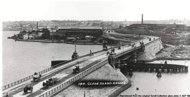
Figure 4 – Glebe Island Bridge, ca1881-1910. (Source: NLA, PIC P803/14/31 LOC Row 64/nla.obj-138926580)
